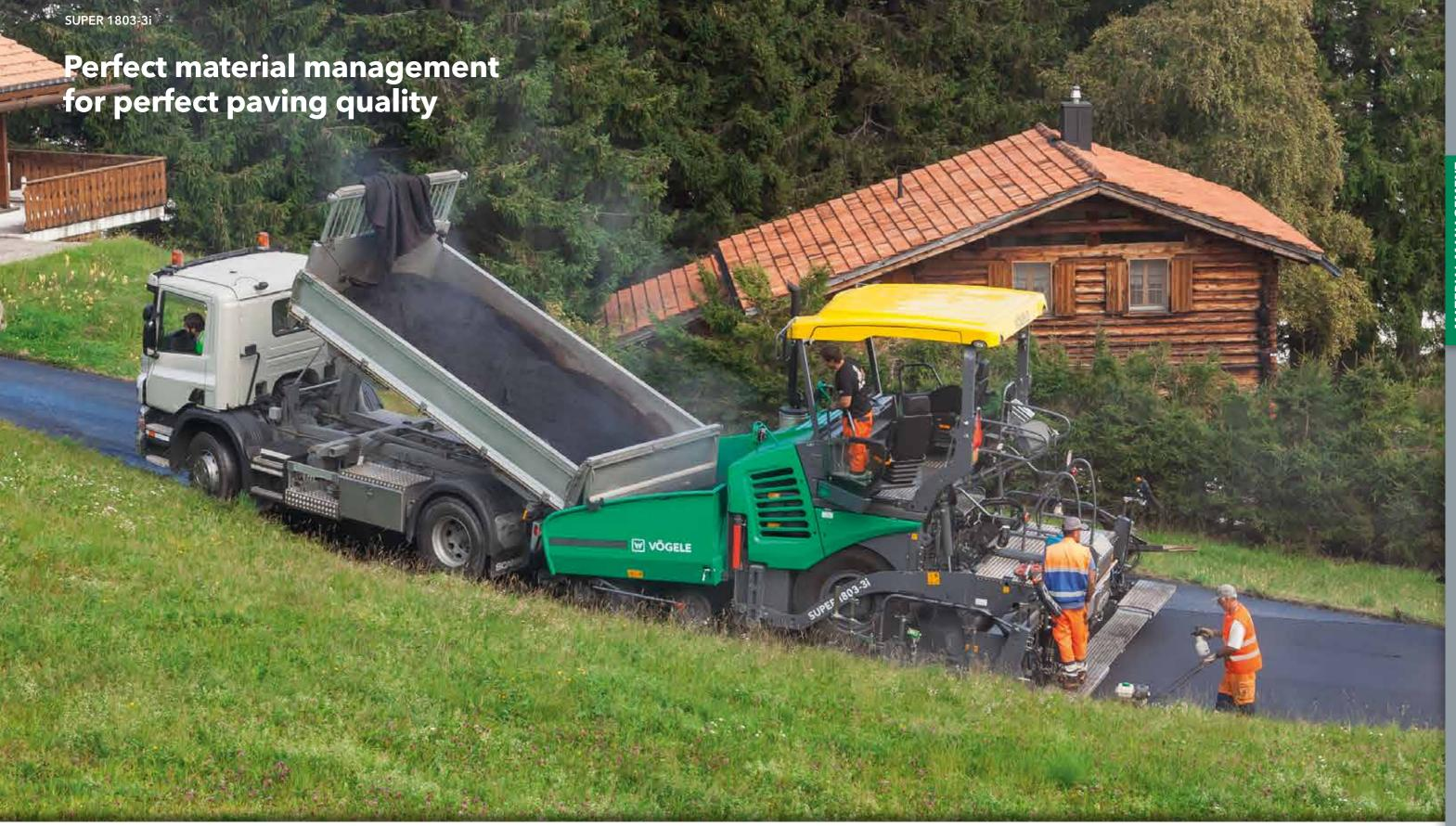
A continuous flow of mix is key to ensuring uninterrupted and high-quality paving. That is why we attach such importance to professional material management when designing our pavers.
