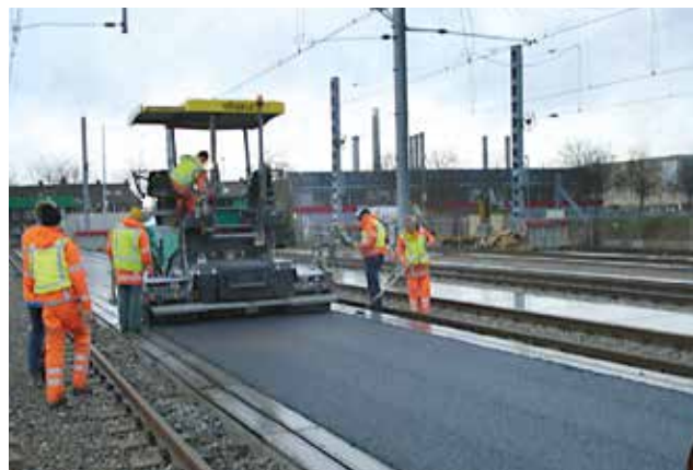
ASPHALT PAVING ON RAILWAY PLATFORMS
