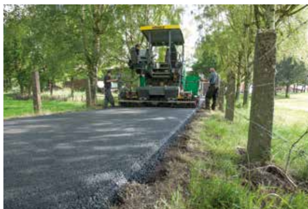
PAVEMENT REHABILITATION ON ACCESS ROADS
